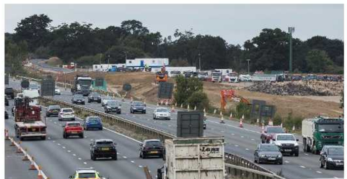
Works and traffic management underway on the M4
